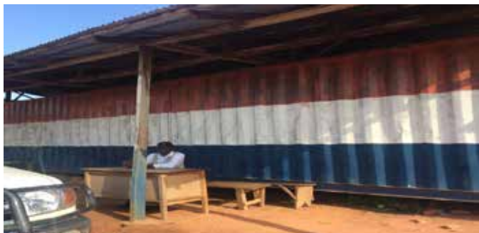
Abandoned Container Warehouse
