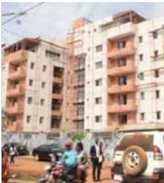
Residential Building under construction in Sinkor
