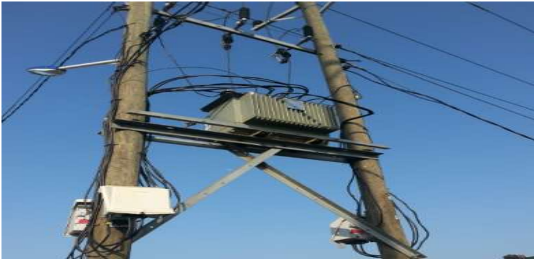
Figure 2: pole-mount single phase distribution transformer
