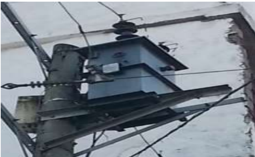
Figure 2: pole-mount single phase distribution transformer
